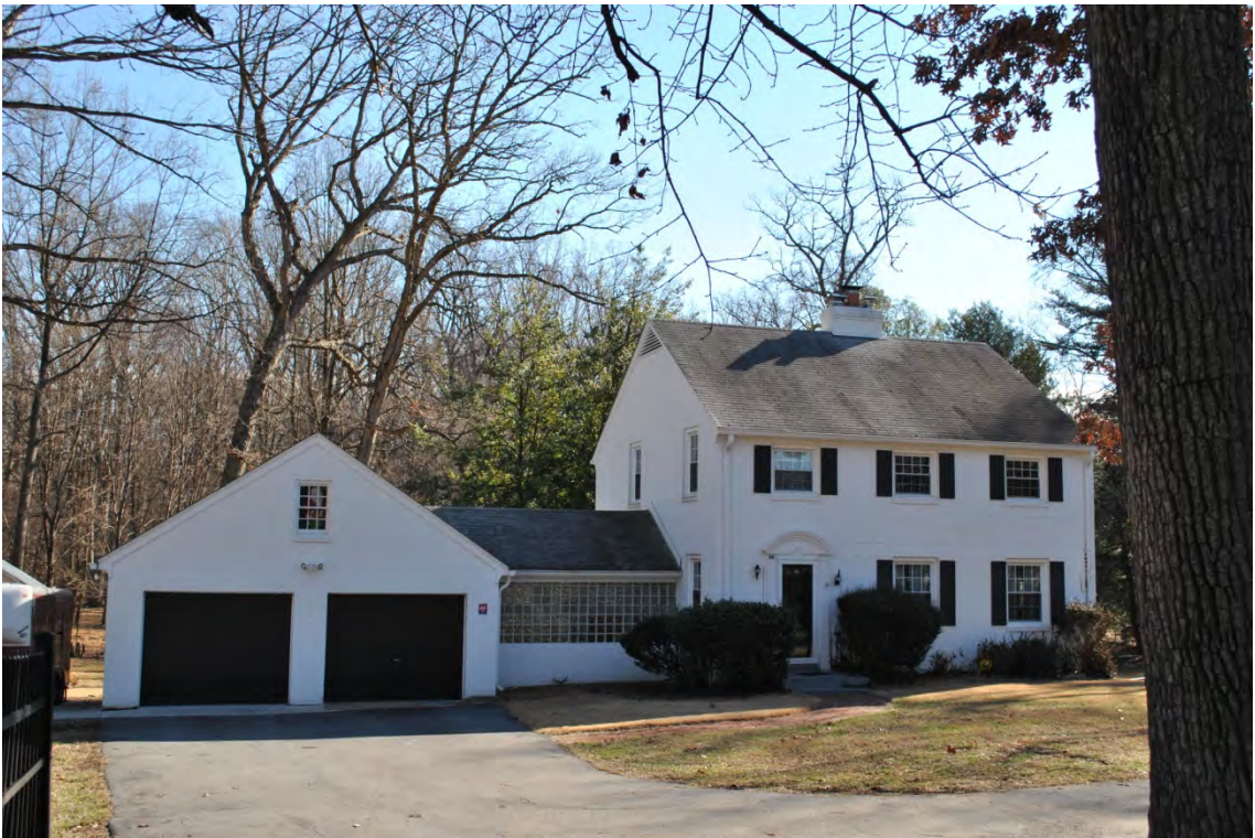
View south at 899 Quince Orchard Road
