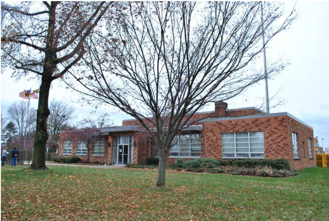
View southwest at the façade of the main and oldest building of the State Highway Administration Maintenance Facility – Gaithersburg Shop
