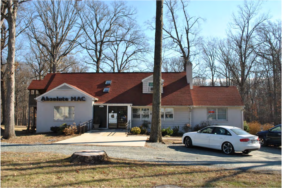
View east at 895 Quince Orchard Road
