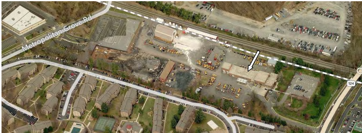
View north at the State Highway Administration Maintenance Facility – Gaithersburg Shop with an arrow points to the main and oldest building on the complex (image from Bing.com)
